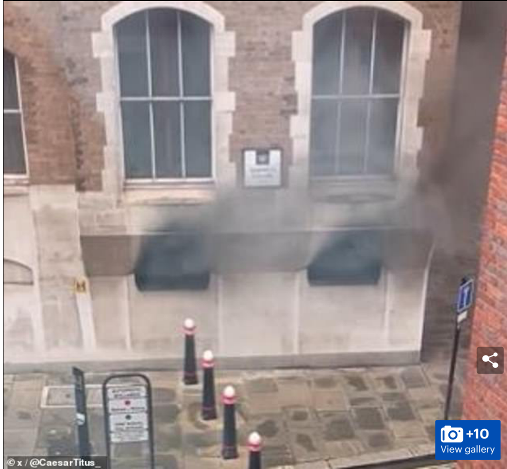
Fire crews had to check out 'multiple buildings' on Warwick Lane
